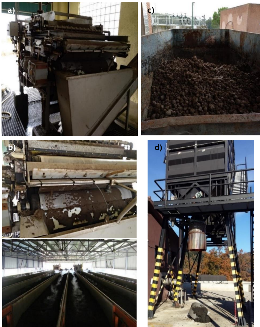
Figure 3-4. Secondary sludge dewatering through belt filter (a and b) and sludge storage in WWTP of Navàs (c). hopper for sludge storage in WWTP of Olot before composting plant (d), composting windrows of composting plant of Aigües de Manresa.
