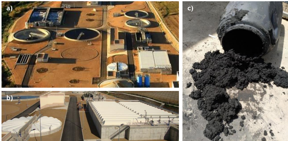
Figure 3-3. Almendralejo WWTP (a and b) and primary sludge equivalent obtained for biodrying.
