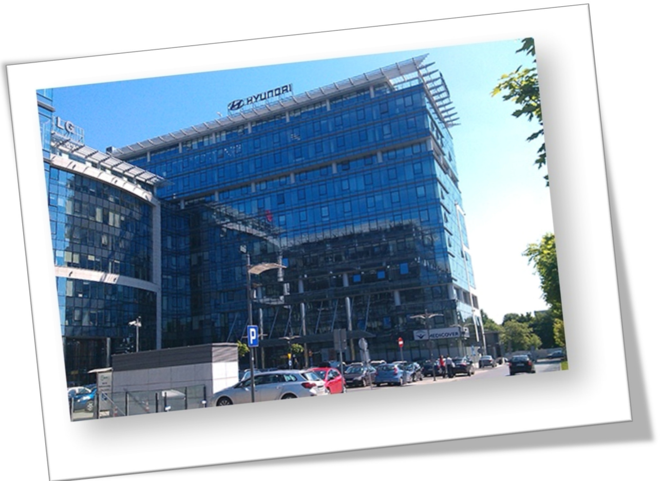
Picture 4-III. View of Warsaw office. Picture by Karolina Woźniak
